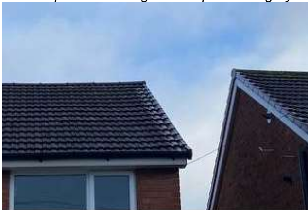
A typical example of a 45 degree roof pitch with grey roof tiles
